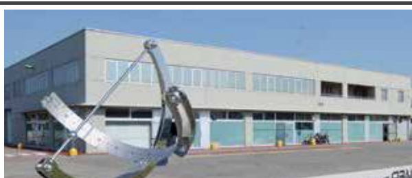
REMER ENGINEERING 1 high-tech production, R&D.
